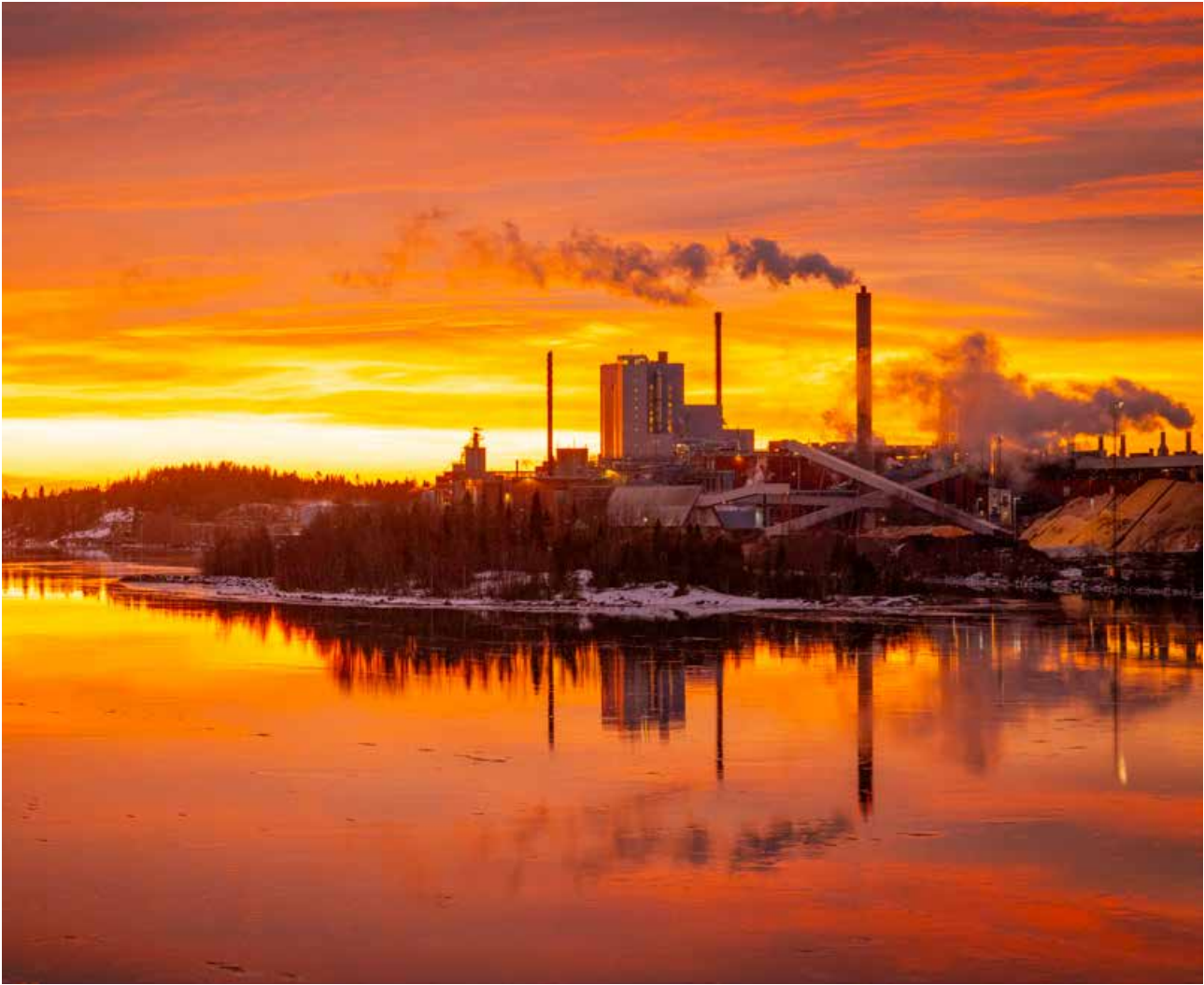
SCA is expanding its kraftliner production at the Obbola paper mill.
