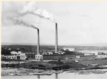
The first decision taken by the SCA Board was to invest in a new kraft pulp mill. The Östrand pulp mill was taken into operation in 1932 and was then, as it still is, the largest production line for bleached softwood kraft pulp in the world.
