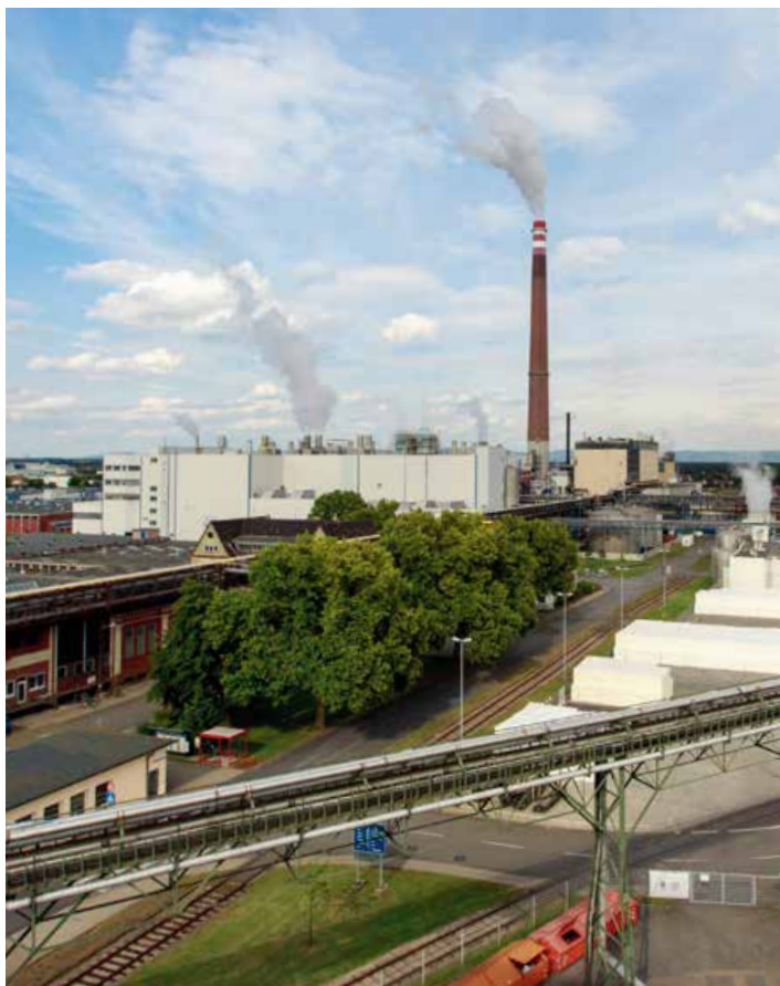
SCA's upgrade of the biogas plant in Mannheim will reduce carbon emissions and increase production efficiency.
