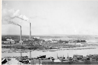
SCA invested in new kraft pulp production with the construction of the Östrand pulp mill
