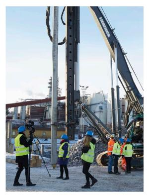
Work on the Östrand project began in February 2016 with a 12 meter concrete pile being driven into the ground.
